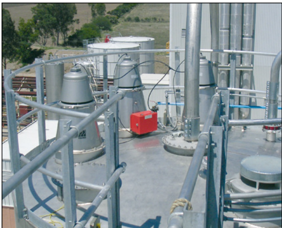
Stainless steel modular bin vents
