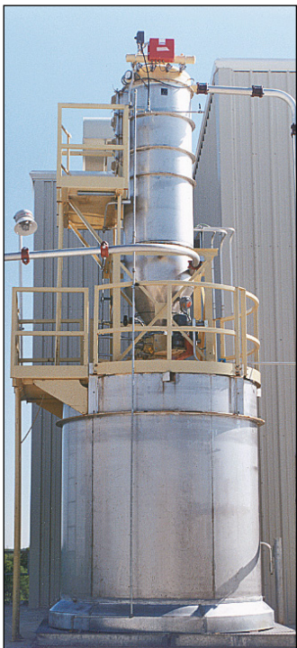
Stainless steel filter receiver
